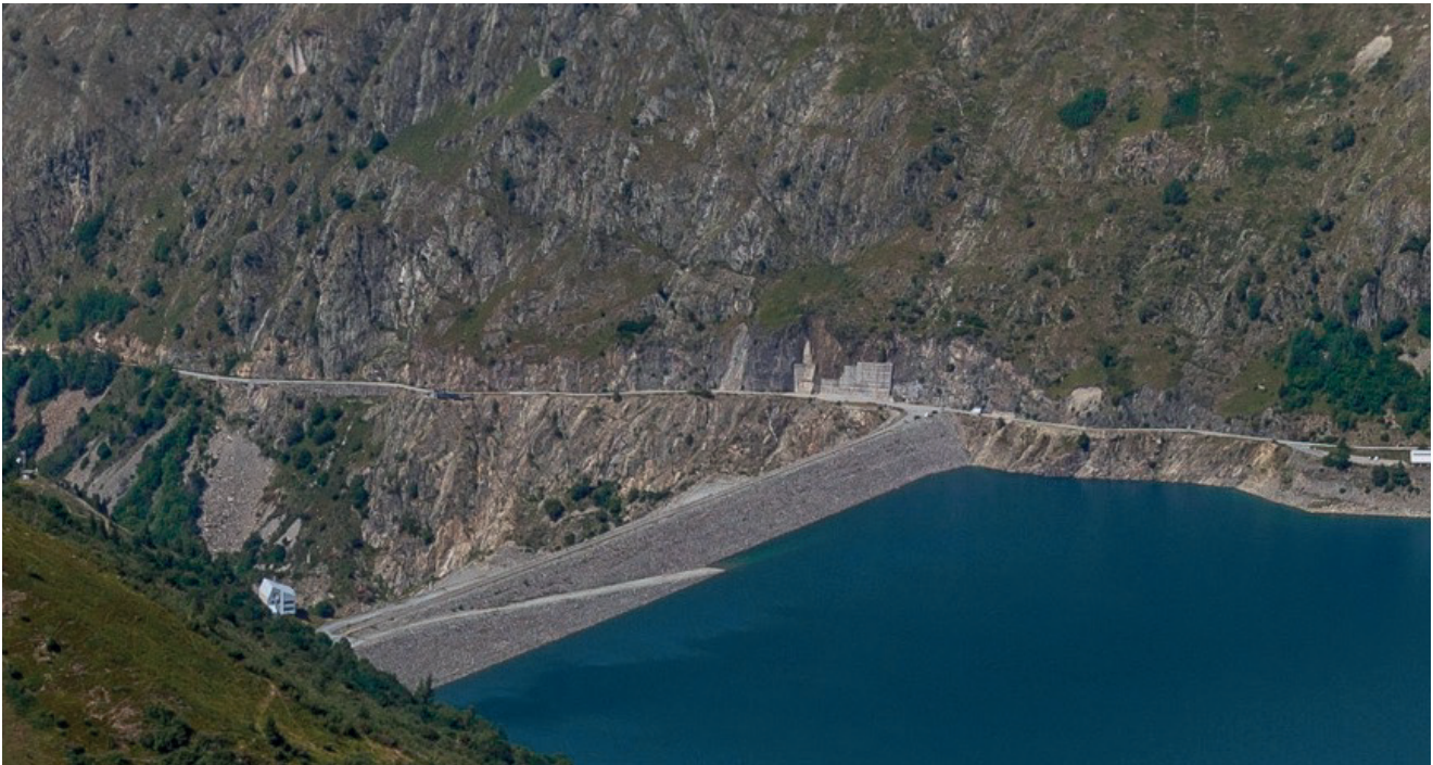
Upper reservoir of the Grand'Maison pumped-storage hydropower scheme in Isère, SE France
