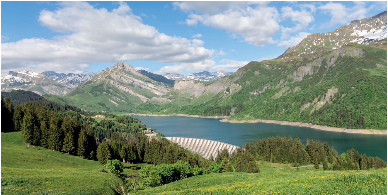
Roselend Dam. France P.
