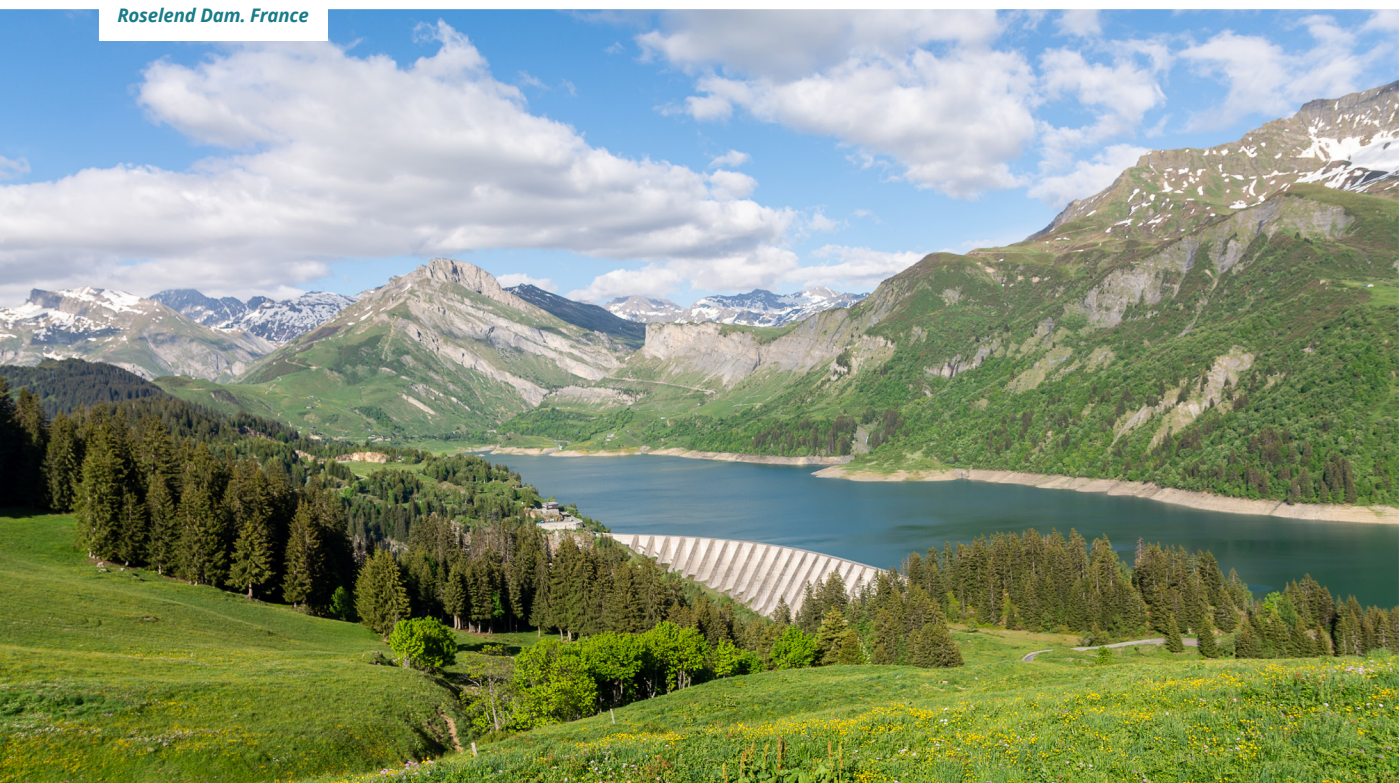
Roselend Dam. France
