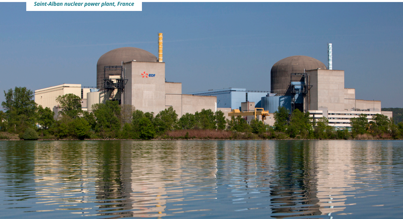
Saint-Alban nuclear power plant, France
